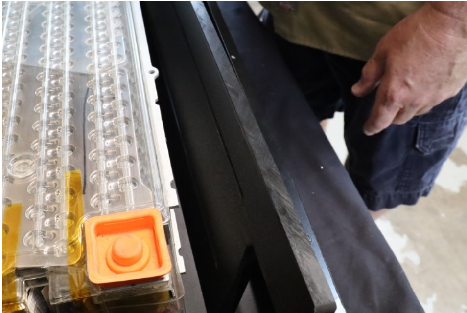
Install front ABS spacer
