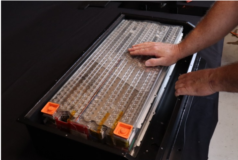
Install second battery module
