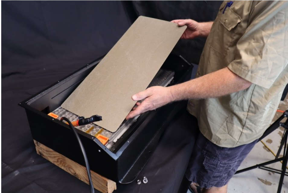
Insert mica sheet on top of lower battery
