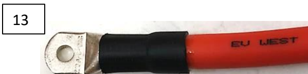
Finish view of a quality installation
